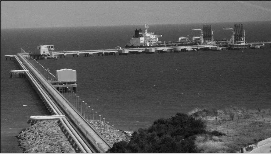
Fig. 1-6. Loading a tanker at a marine export facility
