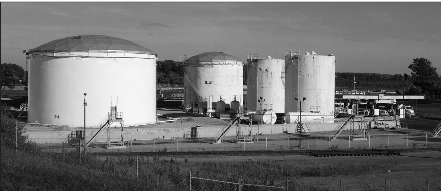
Fig. 1-7. Refined products terminal. The storage tanks are shown on the left, and the truck loading rack is shown on the far right.
