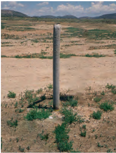
Figure 2.22. Cahn Gas Com 1 Abandonment Marker (Original photo)
