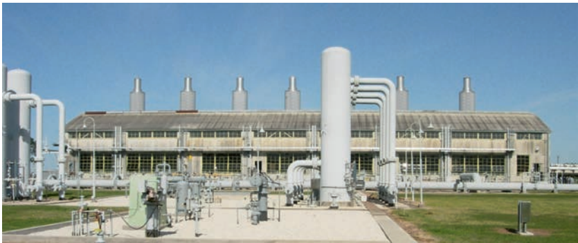
Fig. 6-8. Origination gas compressor station near Victoria, TX. Several gathering lines from onshore and one from offshore enter this mainline origination compression station. The natural gas is aggregated into a common suction header and a combination of the seven reciprocating compressors, driven by natural gas-fired reciprocating engines, adding pressure to the gas before it is discharged into a 30-inch natural gas mainline. Courtesy Williams Gas Pipeline.
