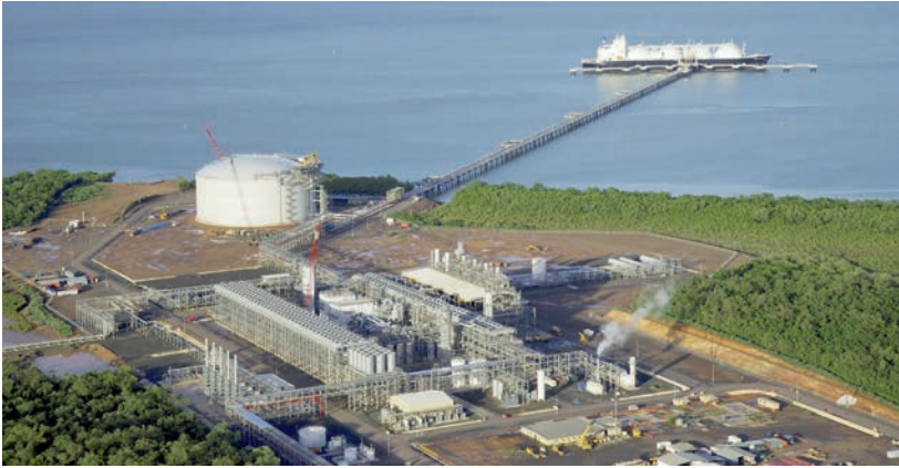
Fig. 6-7. LNG or liquefaction export facility. The facilities in the foreground liquefy the gas by refrigeration. The domed tank stores the LNG until it is loaded on the ship in the background. Courtesy ConocoPhillips.
