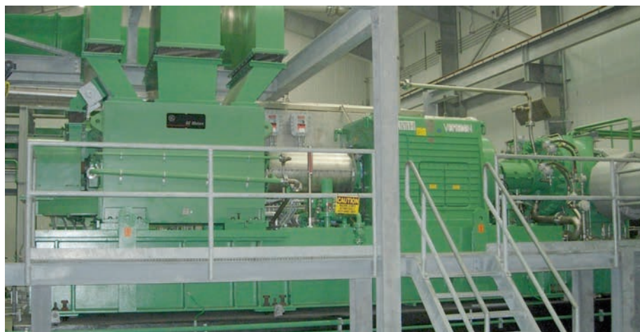
Fig. 6–10. Inside a booster station with centrifugal compressors. Electric motors, not gas-driven engines, are often used in stations to meet emission standards. In addition, the station may be insulated for noise reduction. The electric motor is on the left, with a variable speed drive; the compressor is connected to it on the right. Courtesy Williams Gas Pipeline.
