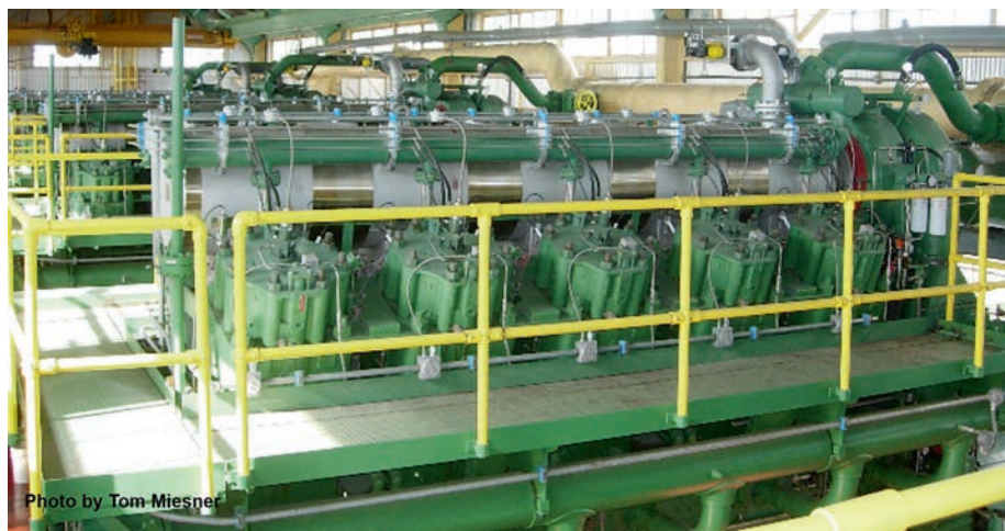
Fig. 6–9. Inside an origination station with positive displacement compressors. From a catwalk about ten feet above the floor in the compressor station shown in Fig 6-10, five cylinders of the V-10 engine are visible. Courtesy Williams Gas Pipeline.
