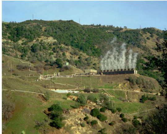
Figure 8-1: The Geysers geothermal complex in northern California. The geothermal resource is excellent at the location, but the topography presents challenges for electric power generation and transmission infrastructure. Credit: National Renewable Energy Laboratory/David Parsons.
